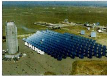
Aerial view of the New Mexico facility. The Cherenkov light collected by 64 heliostats in the array of 200 is concentrated onto photomultiplier tubes in the tower.
